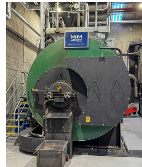
AlSCO Uniforms Christchurch, New Zealand Branch - Biomass Boiler
